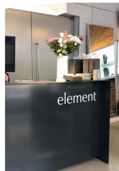
Flood recoverable counter and in the background the interior doors are now 'Rainscreen' panels.
