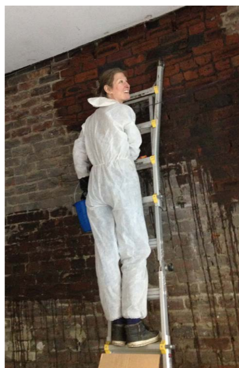
Brick wall cleaning. Some walls were left as bare brick, and sealed.
