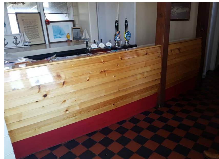
The bar is made of marine ply.
