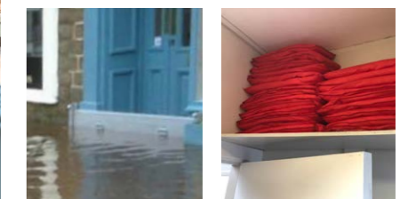
A robust 'slot in steel barrier' is fitted before a flood.
