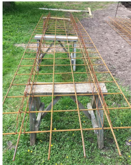
Cut the 'chairs' and mesh to size then tie the chairs to the bottom mesh sheet. . Then tie the top sheet to the top of the chairs forming a cage like structure.
