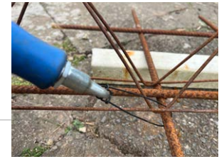
Tying the rebar with the Draper twister tool
