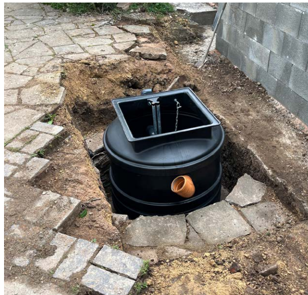
Sump in place ready for concrete
