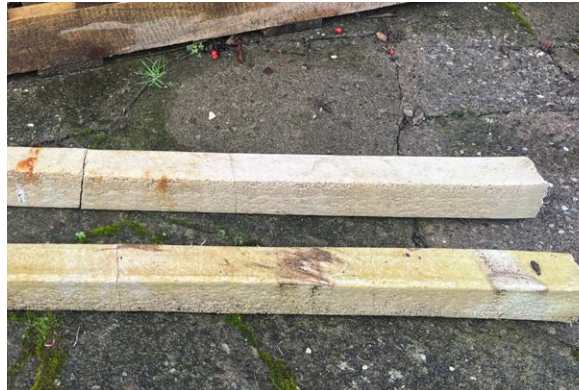
Mars Bars to rest the cages on in the foundation
