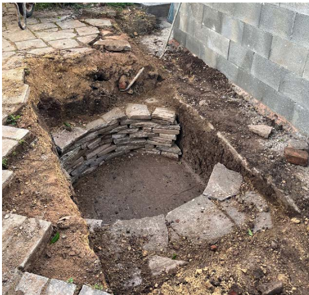
The paving slab 'well'
