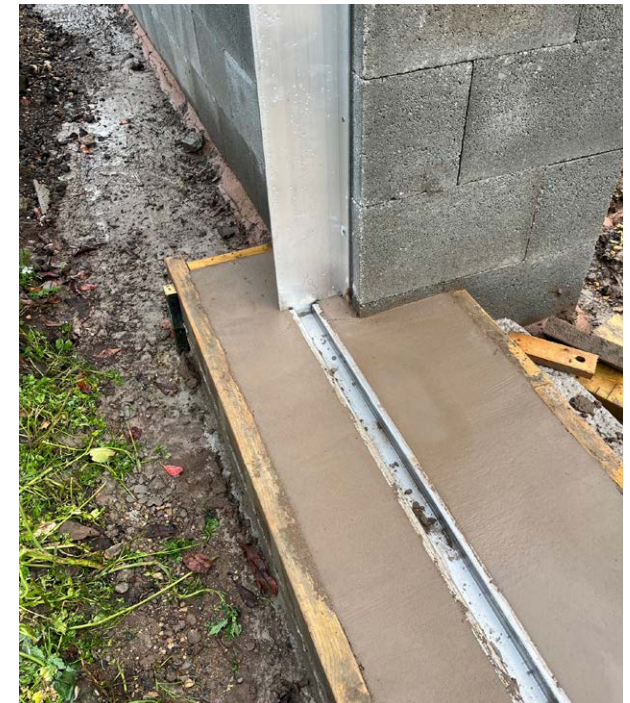
The lower part of these brackets would be embedded in the sand/cement mix that made-up the sill of the opening.
