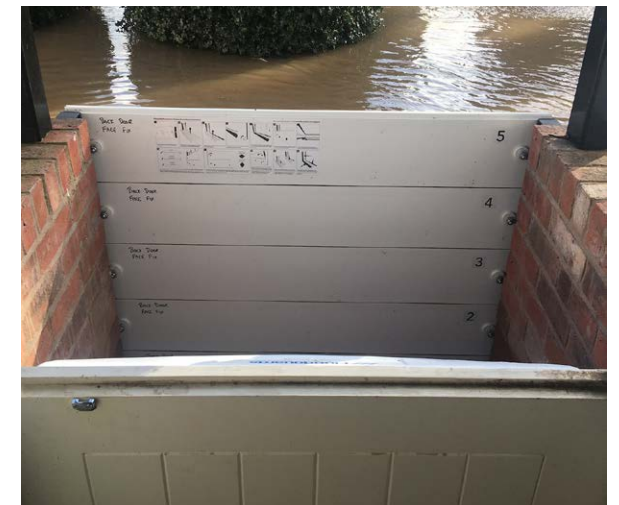
Puddle pumps are placed between the two sets of barriers which manages any water ingress into the porch.
