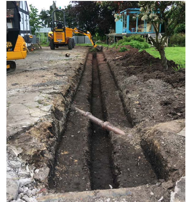
Centre trench excavated
