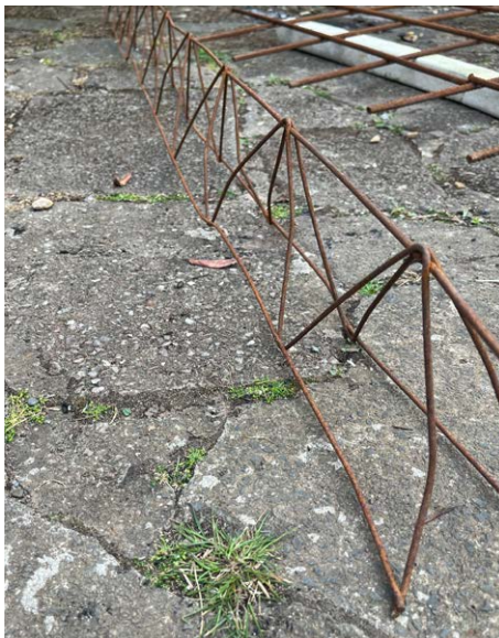
Cut the 'chairs' and mesh to size then tie the chairs to the bottom mesh sheet. . Then tie the top sheet to the top of the chairs forming a cage like structure.
