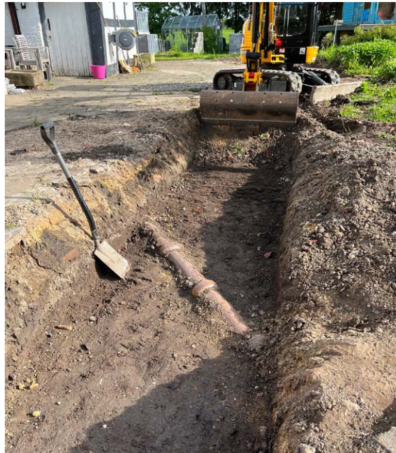
Initial foundation dig
