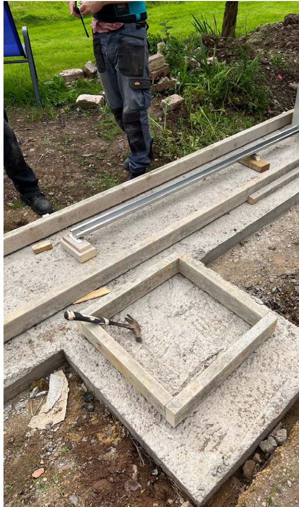
The lower part of these brackets would be embedded in the sand/cement mix that made-up the sill of the opening.
