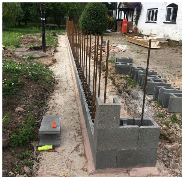
Second and third courses dry laid
