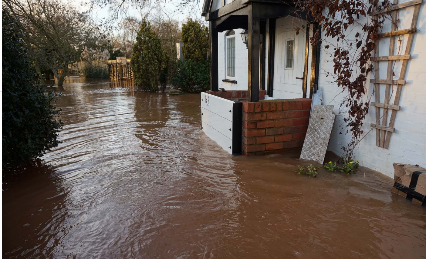
Secondary flood barriers have been fitted to the front of the porches.
