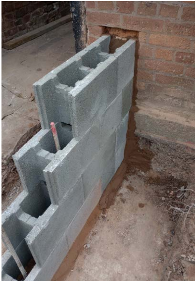
Where the wall joined the garage block it was cut into the existing brickwork to ensure stability and a strong watertight seal.
