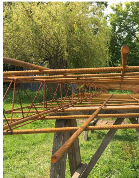
Cut the 'chairs' and mesh to size then tie the chairs to the bottom mesh sheet. . Then tie the top sheet to the top of the chairs forming a cage like structure.
