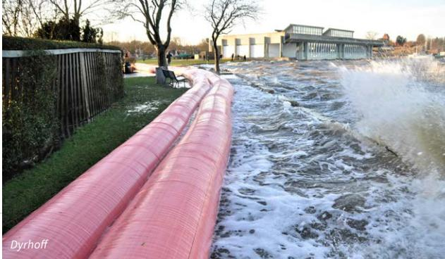
The NoFloods™ water tube barrier is an effective and rapidly deployable flood defence system available in up to 200m long sections and infinitely extendable.
