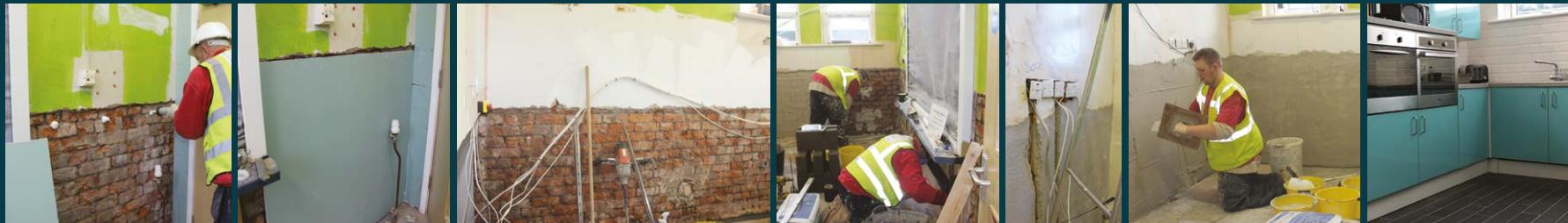
A double-layered replastering system was used, the first was the Dryzone Damp Resistant Plaster Flood System, which is a waterproof and salt retardant plaster, which owing to its porous structure will dry down very quickly should future flooding occur.
