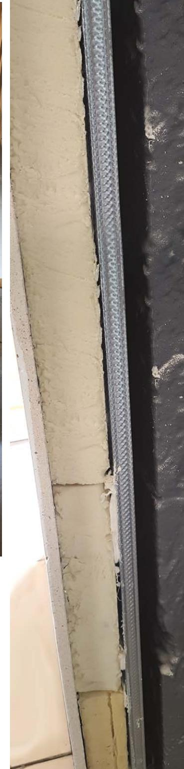
Dragon Board is made from magnesium oxide and magnesium chloride, water and a special fibrous material used for strengthening. It is water resistant so is suitable for floors and walls and can be painted onto with a breathable paint for a finished look.
