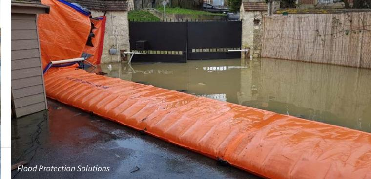
The Water-Gate is a temporary flood barrier which is unique in the way that, once rolled out, it self-deploys. It uses the weight of the water to hold the water back.
