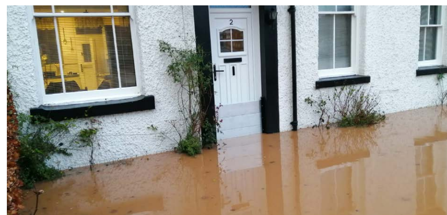
Flood door at the front of the house has a flood barrier as a backup.
