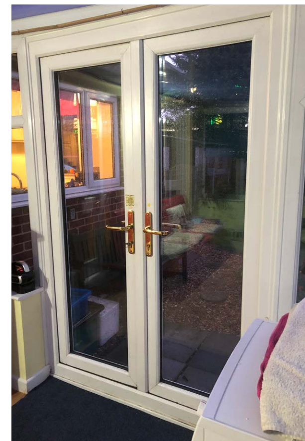
Flood resilient patio doors have been installed.
