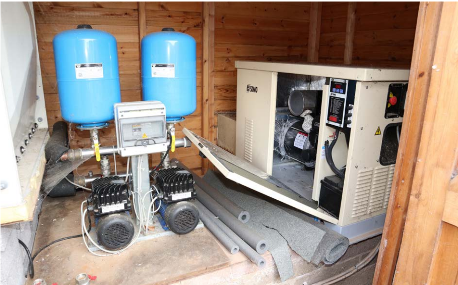
LPG Backup generator, strong enough to run the pumps during a power cut.
