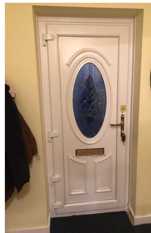
Flood resilient front door has been installed.
