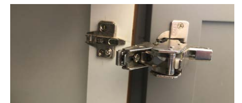
Kitchen doors have easy release hinges, so the doors can be removed quickly.
