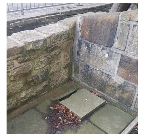
Sump created, into which powerful submersible pump can be dropped when flooding commences.
