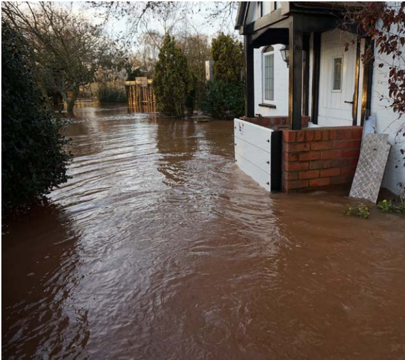
Secondary flood barriers have been fitted to the front of the porches.
