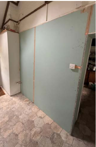
The walls were stripped back to brick, a waterproof membrane installed, moisture resistant plasterboard fitted and skimmed with plaster, allowing the wall to breathe.
