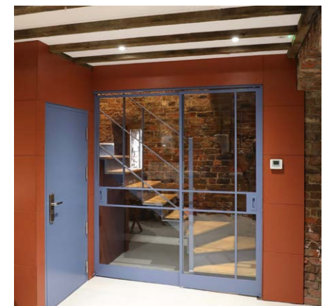
Glazed sliding door/screen in powder-coated steel.
