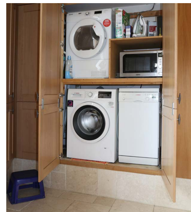
White goods are positioned high up, on a brick-built plinth and are sited inside a cupboard.
