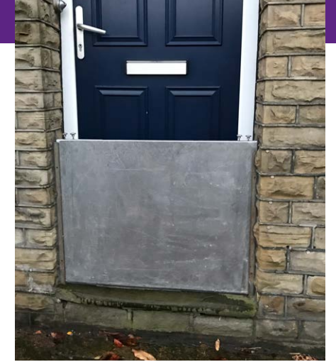
Aluminium slot-in flood barrier.
