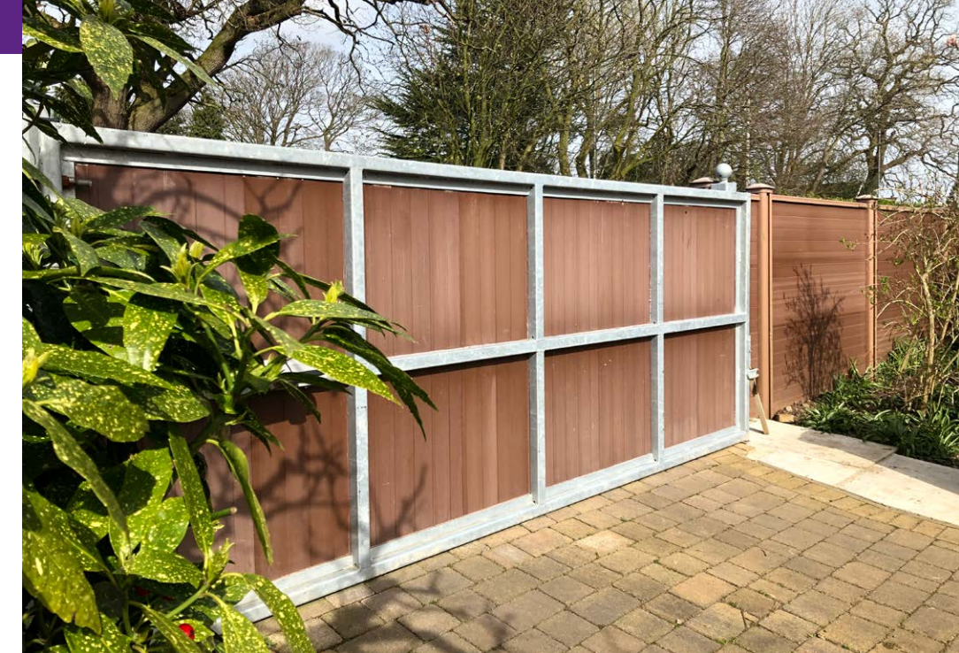
The front entrance gate is the same material as the fence panels and is fitted tightly to prevent ingress of water.
