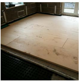
Channels and membranes with sumps and pumps to remove water, then closed cell insulation and finished with removable plastic flooring.
