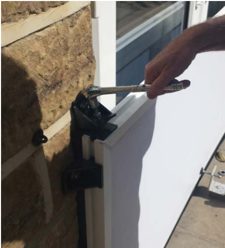
Fitting new taller but lightweight barriers.
