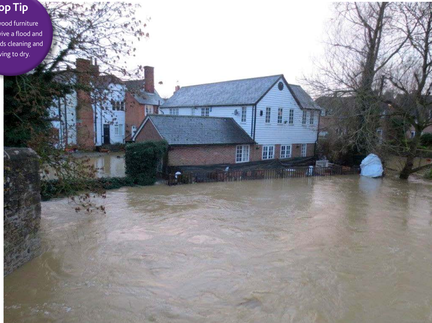
The building skirt system usually coped quite admirably and no water entered the property until it was overtopped in 2013.
