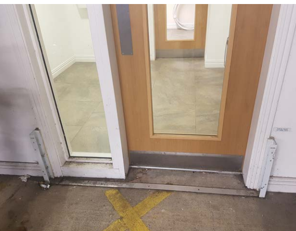
Flood barriers to all doors and UPVC door architraves.
