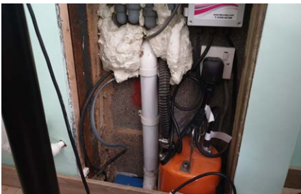
Sub-floor automatic high-performance skimmer pump.
