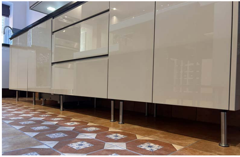
New raised kitchen installed on stainless steel legs.
