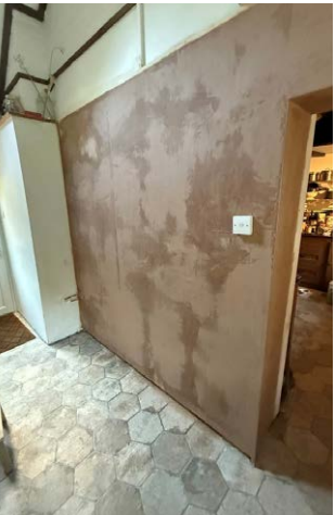
The walls were stripped back to brick, a waterproof membrane installed, moisture resistant plasterboard fitted and skimmed with plaster, allowing the wall to breathe.
