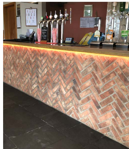
The bar is now brick and has been treated with a waterproof spay. The floor is tiled.
