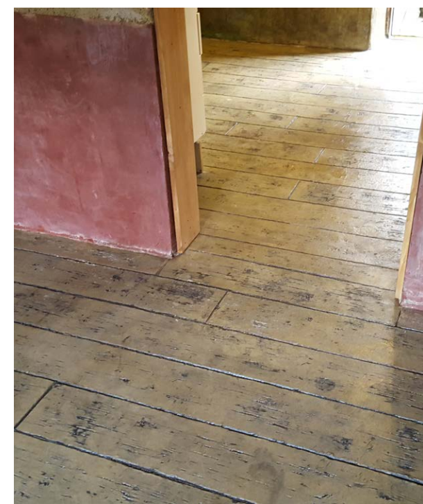
The floor is concrete, with an antique wood effect pattern, and sealed to give a gloss finish.
