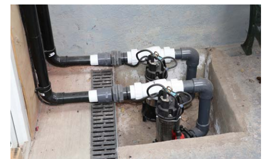
Submersible pumps used at low spots and work well.
