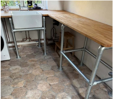
The flooring was stripped back to the concrete base, a liquid damp proof membrane applied, then a further layer of silicone was applied and topped with porcelain tiles. They have also made some modifications to the kitchen to help reduce both the preparation and clean up time.
