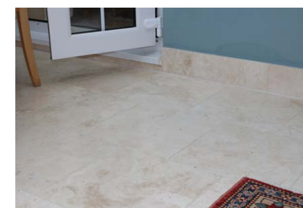
Stone flooring downstairs up to skirting height.
