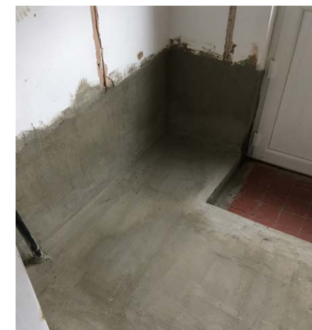
Waterproof slurry was applied to the floor and the walls up to a metre high.
