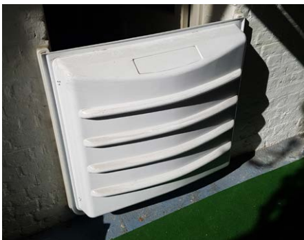
Flood barrier on the back door.
