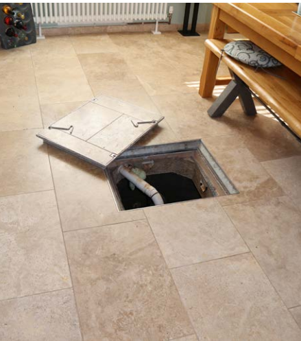
Installed three submersible sump pumps in chambers below the floors, all are interlinked with pipework.
