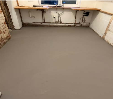
The flooring was stripped back to the concrete base, a liquid damp proof membrane applied, then a further layer of silicone was applied and topped with porcelain tiles. They have also made some modifications to the kitchen to help reduce both the preparation and clean up time.
