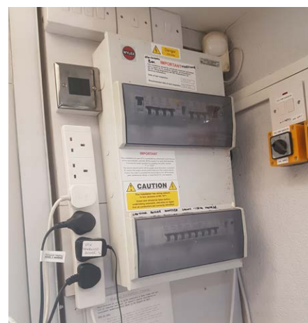
All electric service points are raised above flood level.
