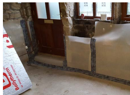
Waterproof membrane during installation.
