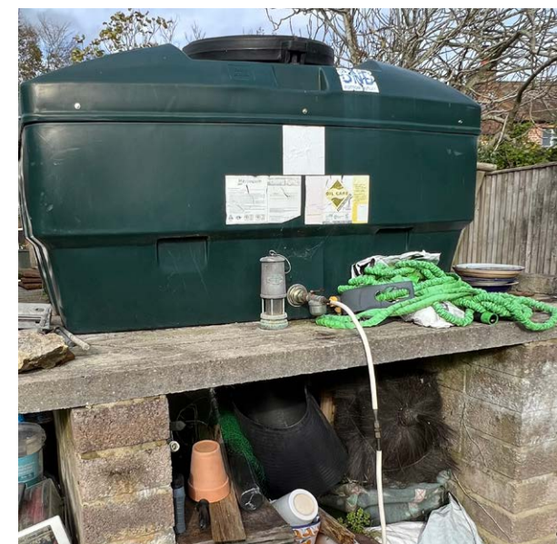
New oil tank was installed on a concrete plinth.
