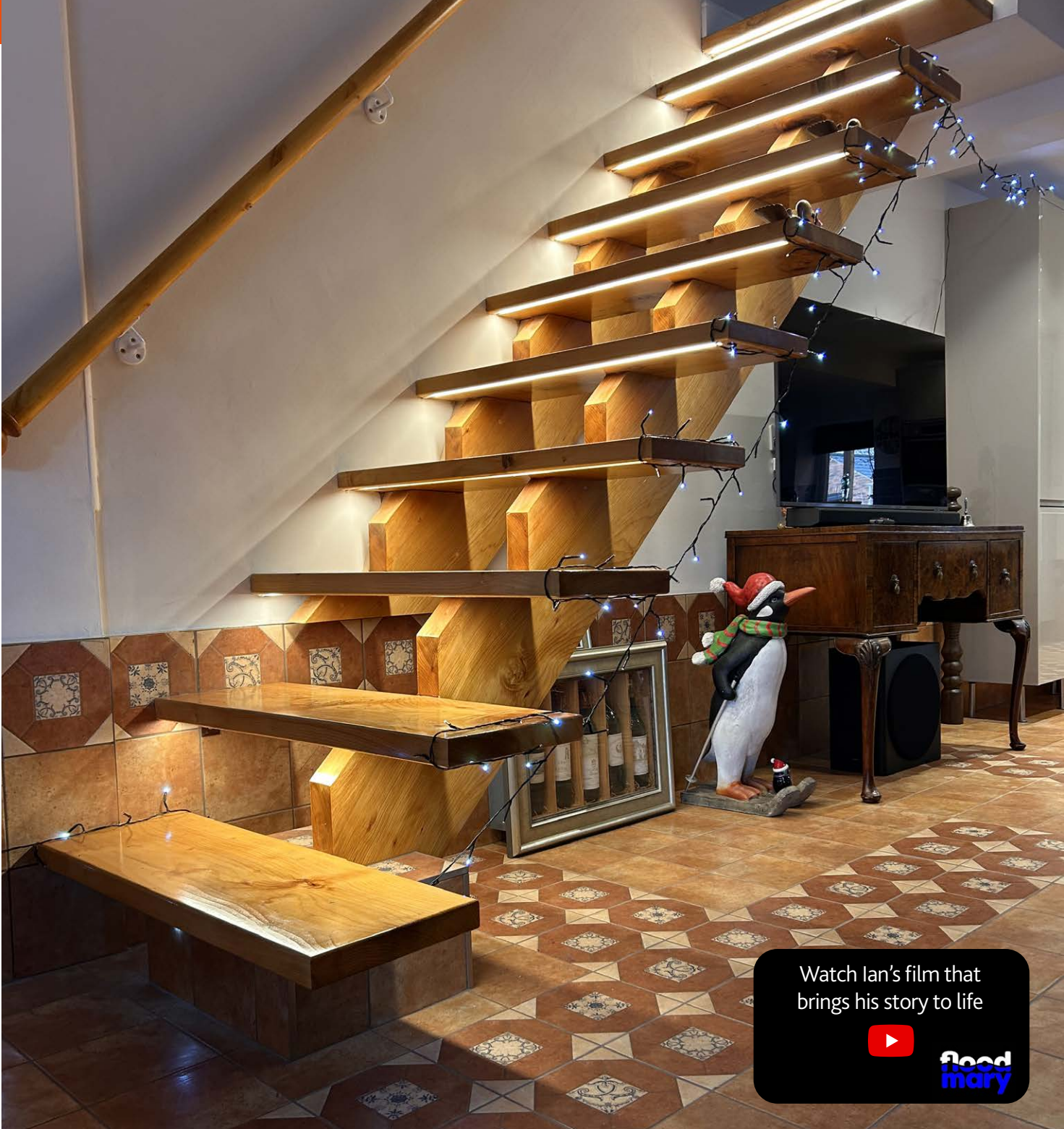
Floor tiles run up the wall to make washing out easier.
