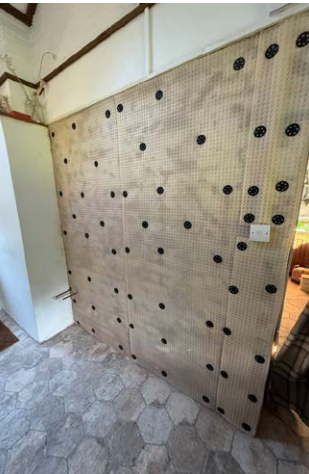
The walls were stripped back to brick, a waterproof membrane installed, moisture resistant plasterboard fitted and skimmed with plaster, allowing the wall to breathe.
