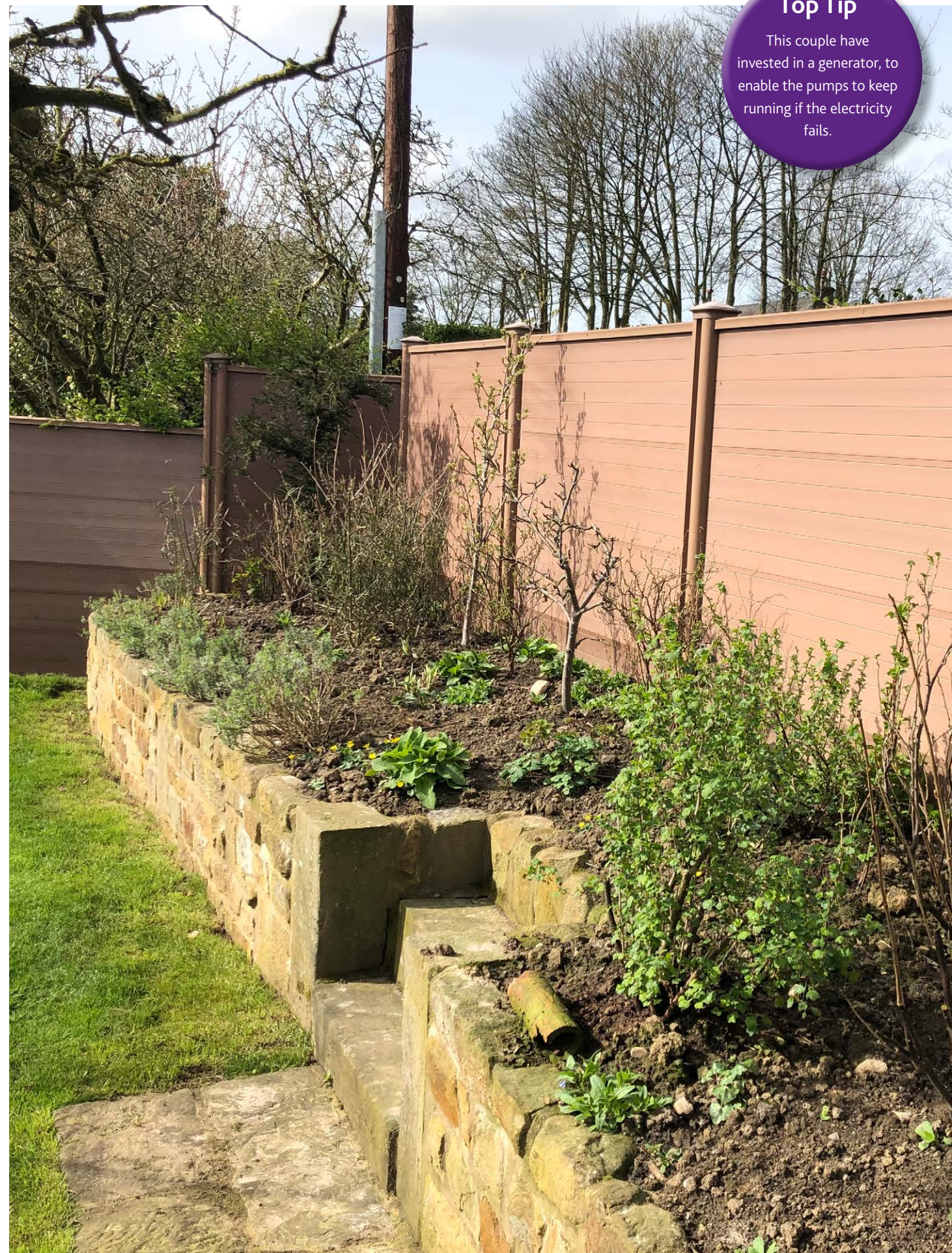
At the perimeter of the garden one-metre-deep holes were filled with concrete, into which posts and reinforced 'Task Green' waterproof fence panels were fitted.
