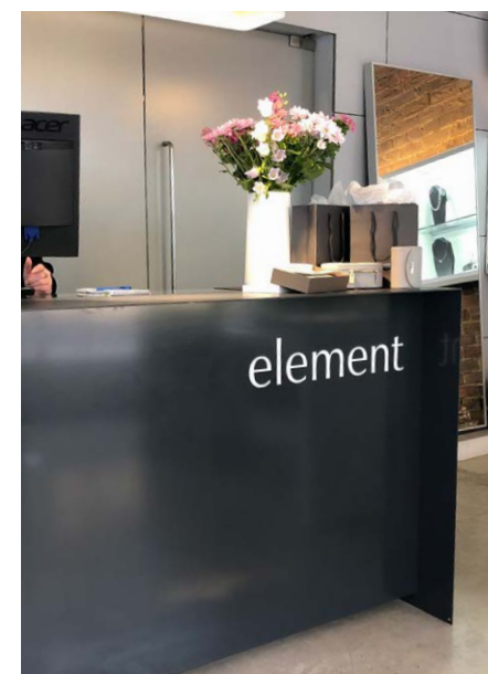
Flood recoverable counter and in the background the interior doors are now 'Rainscreen' panels.
