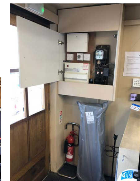
Electric meter and fuse box sited high up.
