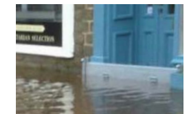
A robust 'slot in steel barrier' is fitted before a flood.
