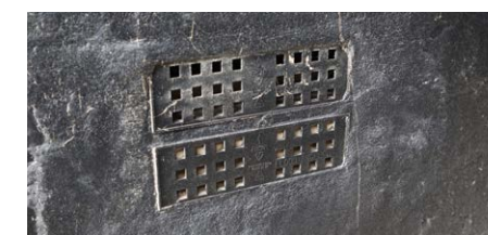
Self-closing airbricks.
