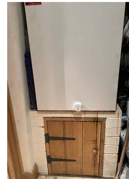
New boiler raised above floor with inbuilt cupboard underneath.
