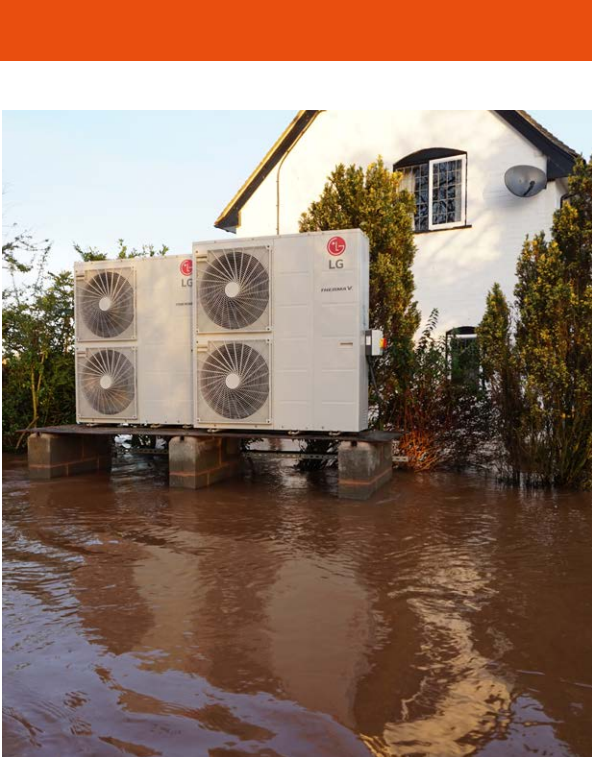
Air source heat pumps have been placed up away from flood risk.
