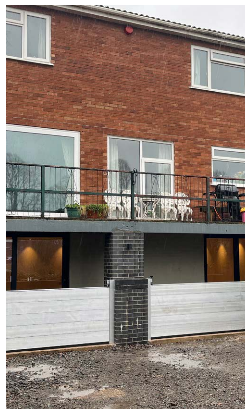
An old brick support pier was completely rebuilt.
