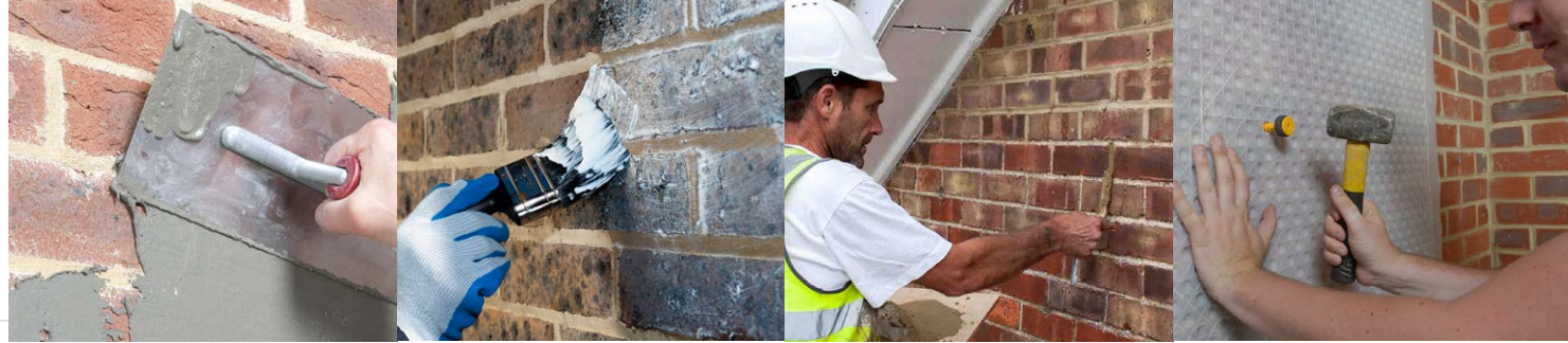
Drybase TS PLUS installation
