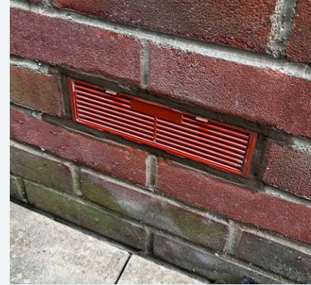
Buffalo Flood Systems
