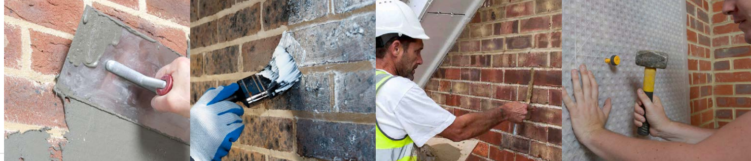
Drybase TS PLUS installation
