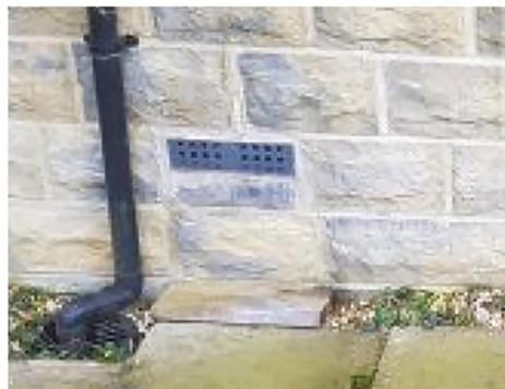
Waterproof render on the bricks and self-closing air bricks to reduce the entry of flood water
