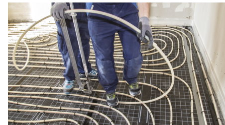
Under floor heating rather than radiators or kick/plinth heaters
