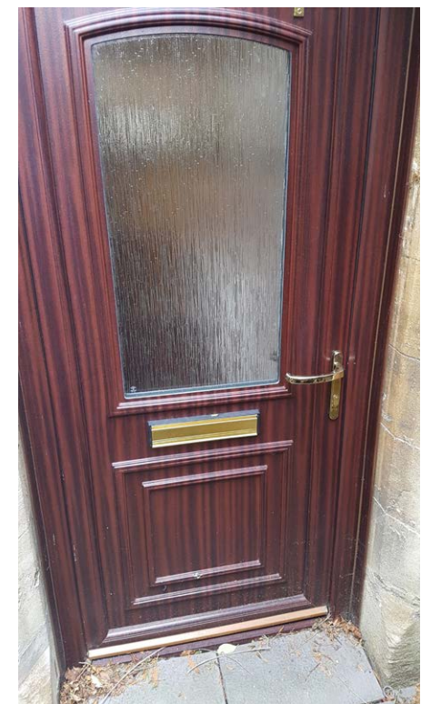
A flood resilient door to the front of the property.
