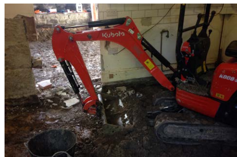
The rebuild involved excavating and 'tanking' the whole of the ground floor
