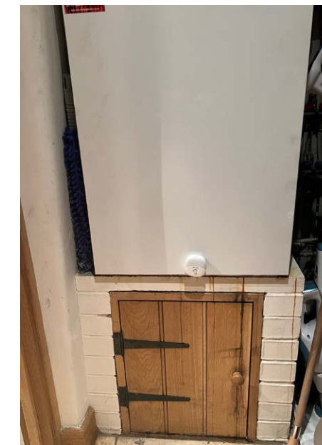
New boiler raised above floor with inbuilt cupboard underneath.
