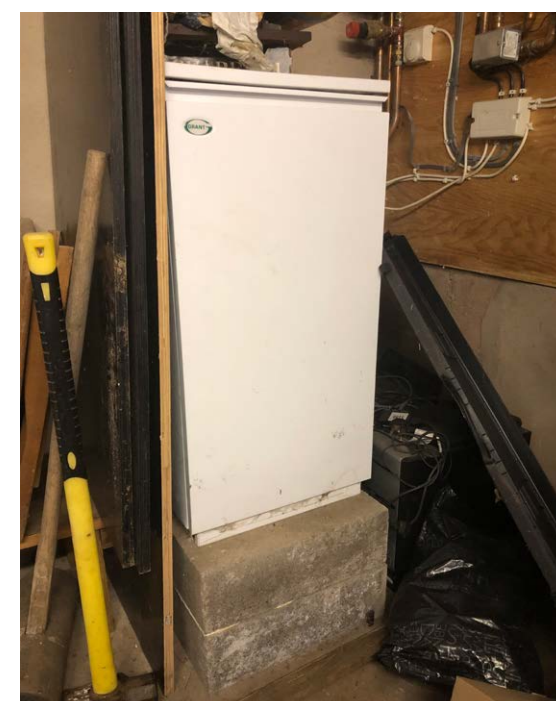
The boiler and freezer raised on a plinth.
