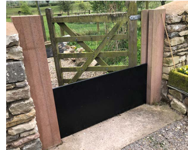
Marine ply slot-in barriers put behind the gates in the wall.
