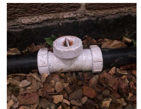
Non-return valve in pipework, to prevent backflow.
