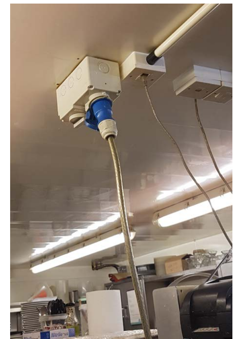
The electricity and gas supply are high up and can be easily turned off and back on.
