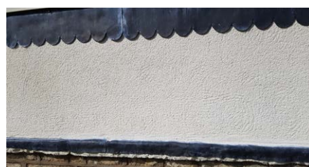
Walls on river-facing side of house have multi-layered waterproofing.
