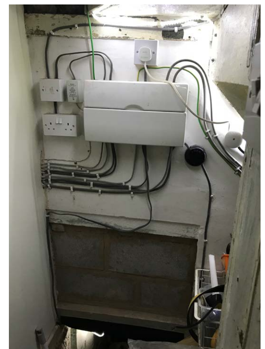
The consumer unit fuse box is still in the cellar but is 1.5m (almost 5') above the floor level.
