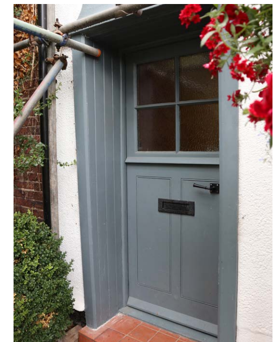
Flood door that is approved for listed buildings.
