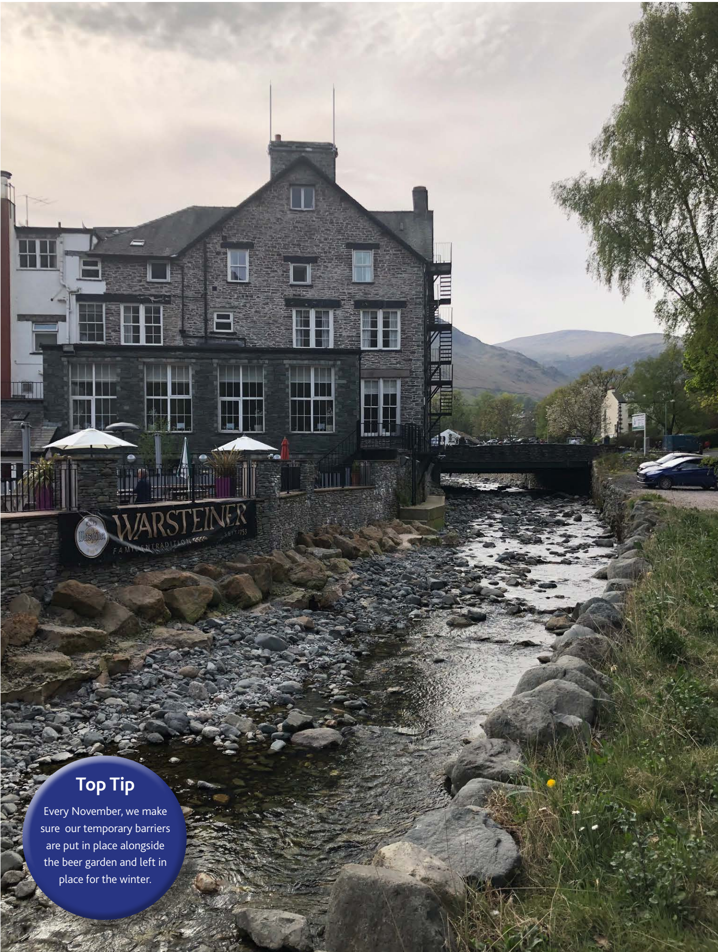
The gable end of the hotel has been strengthened with concrete cladding and large rocks placed in front of it.
