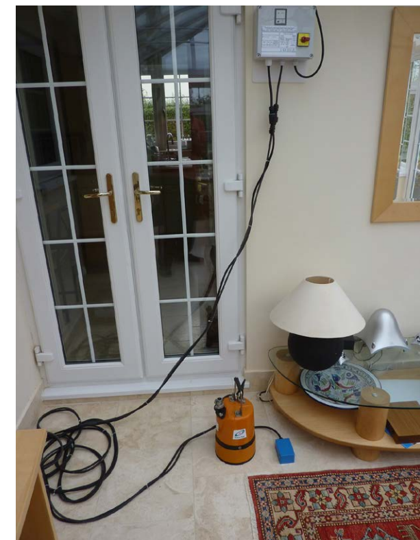
Electrics installed up high, which come down from the floor above, enabling them to run powerful puddle pumps.
