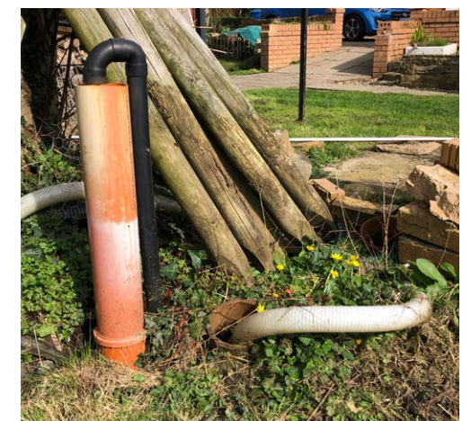
Rainwater runs through a series of French drains into a large sump into which a strong pump is fitted which pumps the water outside the garden boundaries.
