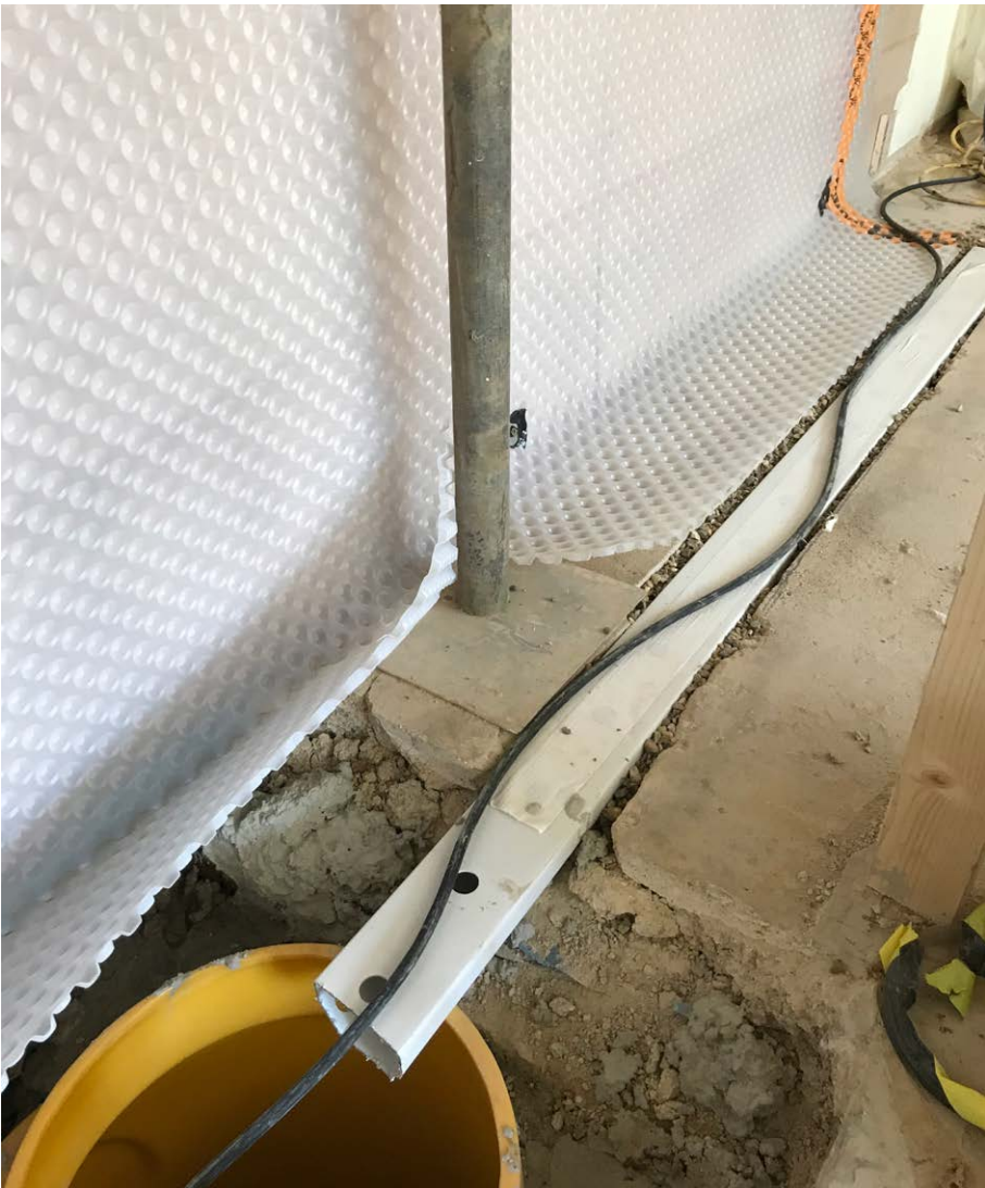
Cavity drainage membrane system and sump pump during installation.
