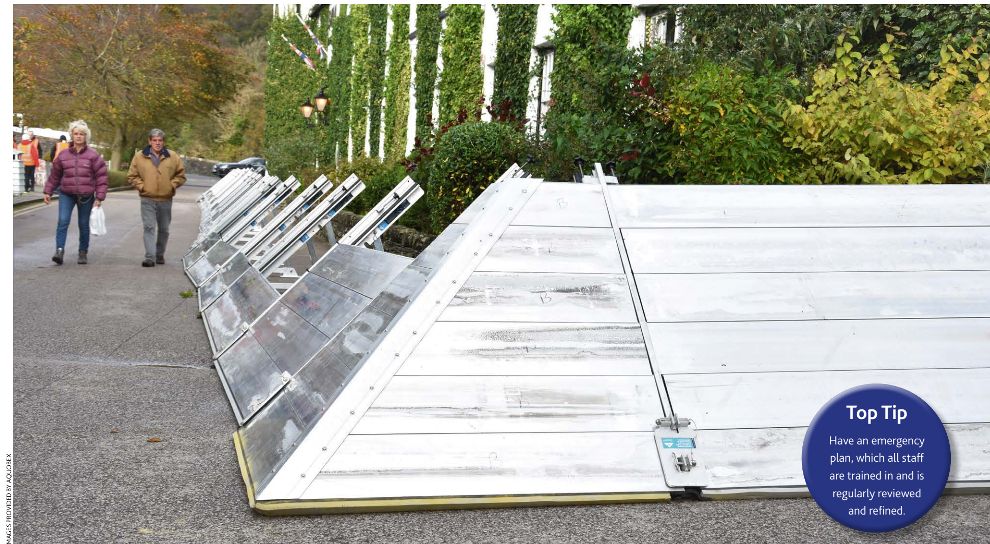
Rigid temporary barriers are installed around the hotel to a height of 1.2m (4'). The hotel has 'Flood Marshals' trained to put the barriers in place, which take 6 people about 1.5 hours.
