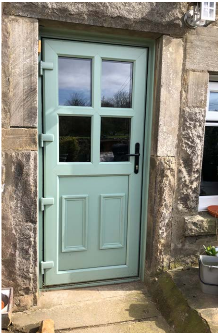
Flood door fitted.
