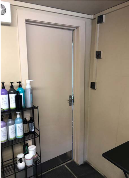
Plastic door architraves and cheap, sacrificial doors.
