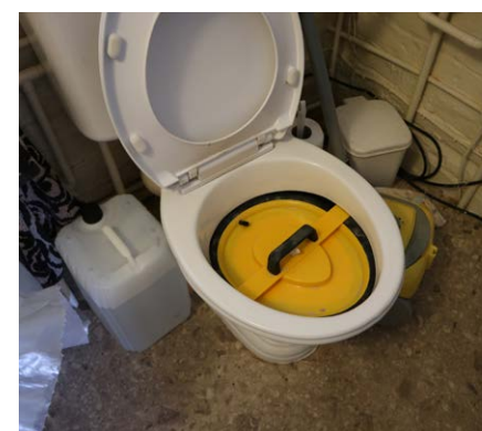
Pan seal as a backup to the non return valves.
