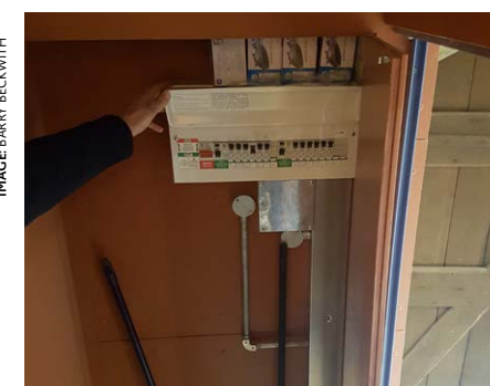
Raised electrics with with drops from ceiling level.
