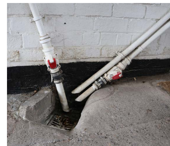
Non return valves fitted to all drainage outlets.
