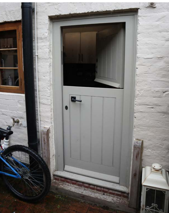
Flood doors, which are approved for listed buildings.
