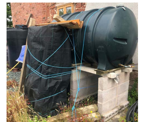
Oil tank housed and secured above highest flood level.
