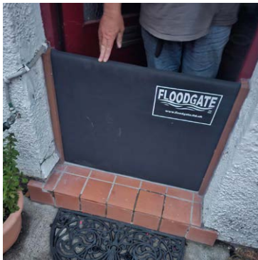
Floodgate - these barriers don't require permanent fixings
